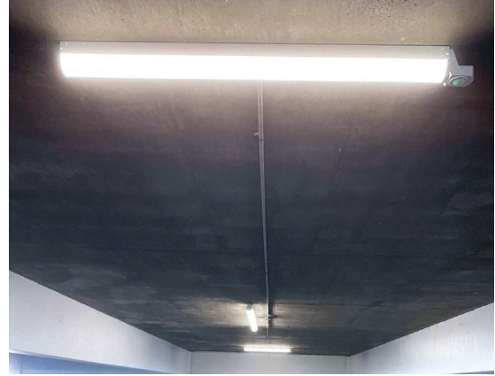
L28500 Series LED Lensed Strips installed in parking garage.
